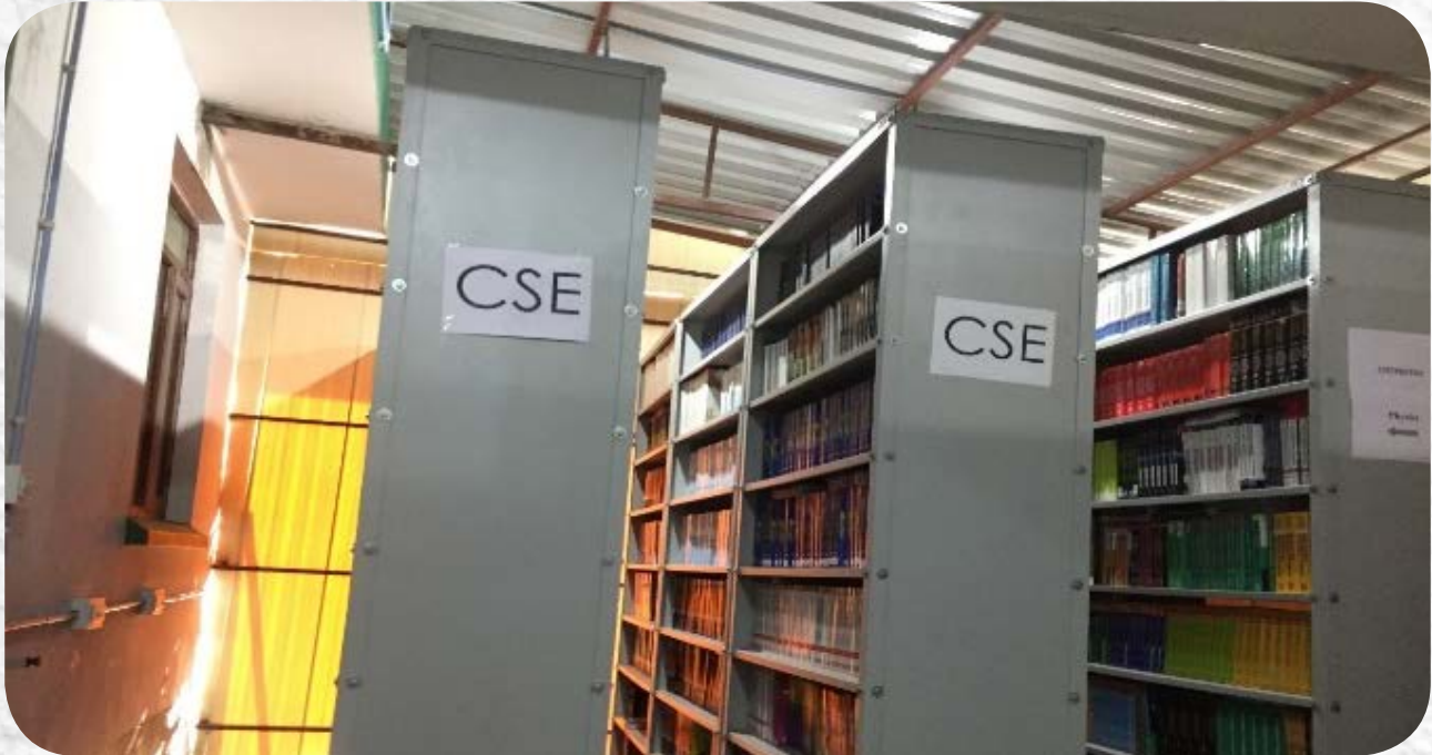
Fig.4 Fabrication of Shed for providing additional space for the Central Library
